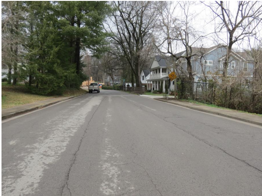
VIEW LOOKING NORTH ON CRAIG AVE.
