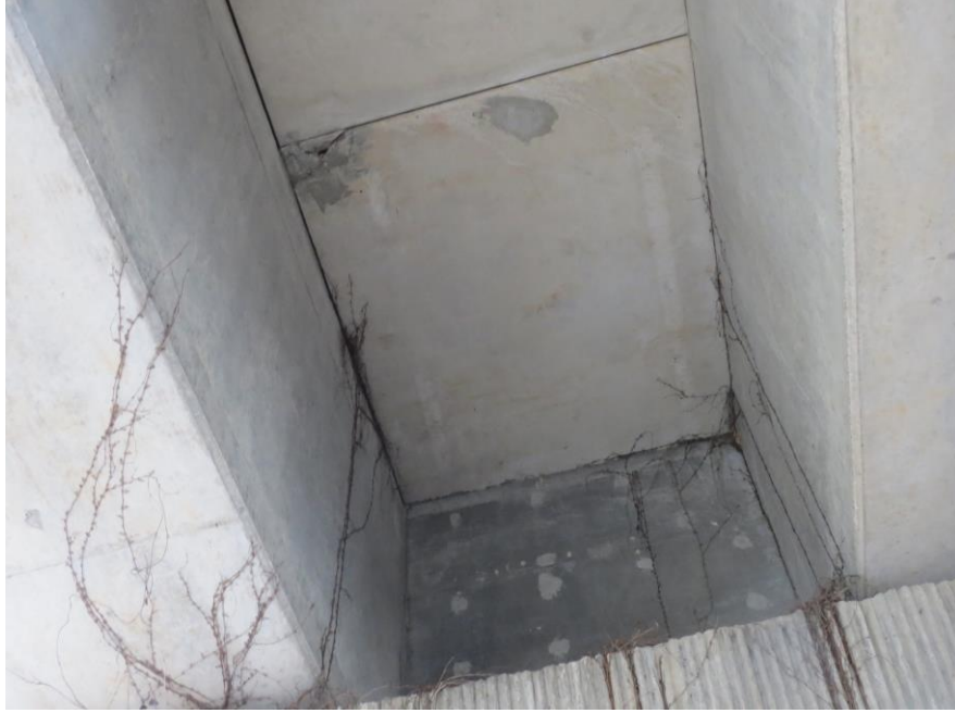
DECK PANEL BAY "A" ABUT. #2 OVERALL VIEW
