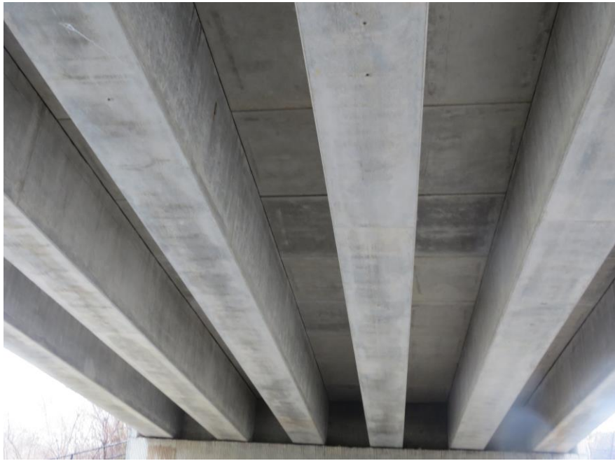
BOTTOM OF DECK
