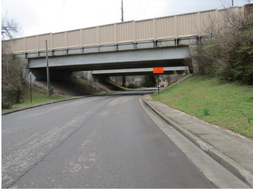
CLEARANCE VIEW RT. SIDE
