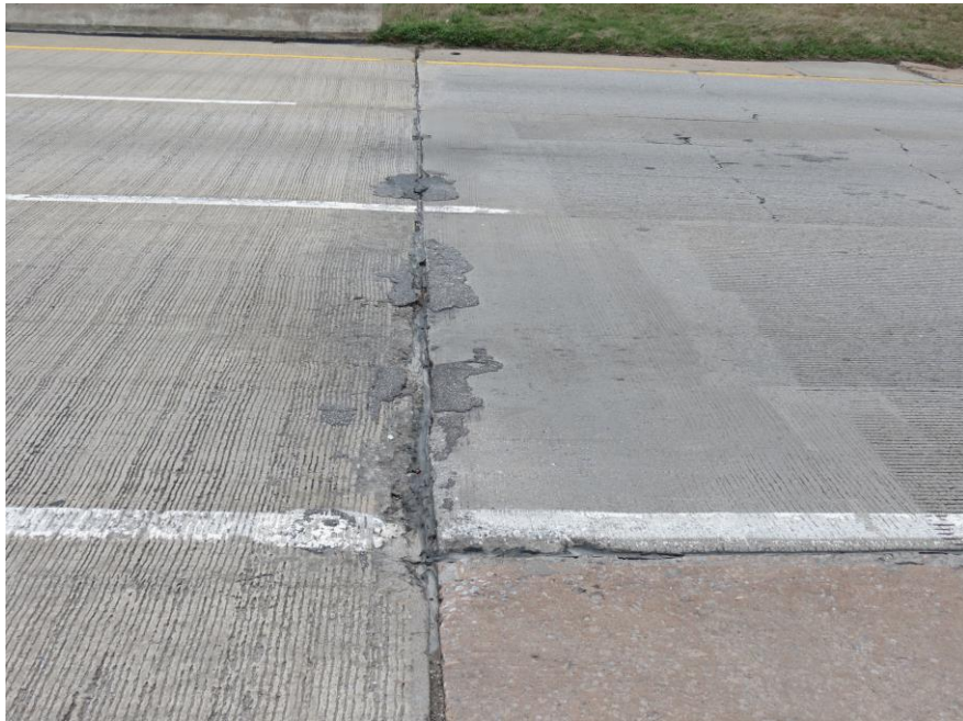
APPR. "B" END JOINT W/ PATCHES EBL
